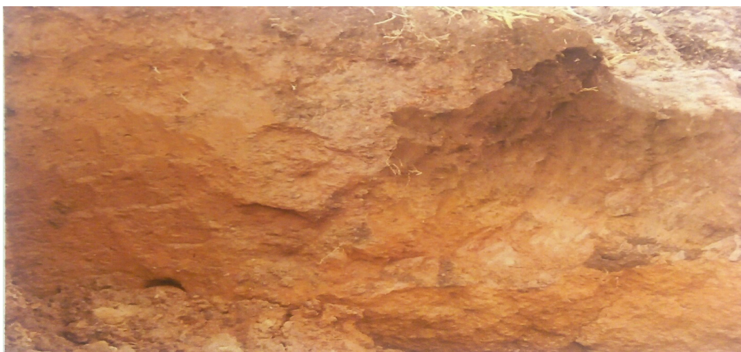
Plate 3. Land degradation as a result of Collapse of Mining Walls at Yelwa Mining site
