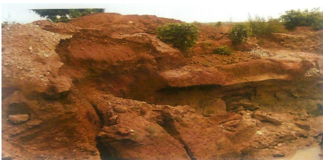
Plate 4. Collapse of Walls in a Baryte Mining Pit in Didango, Karim Lamido LGA
